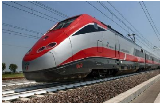
High Speed/High Capacity Rail Infrastructures
